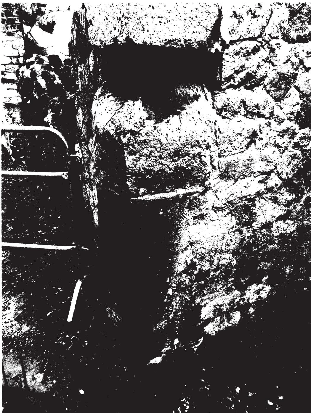
**Figura 9 PARETE OVEST-AMBIENTE 9: BLOCCO IN TUFO DELLO STIPITE DA INTEGRARE**
